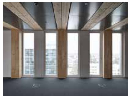
Ceiling panel to conceal systems at LCT ONE Photo credit: Martinsons Byggsystem
