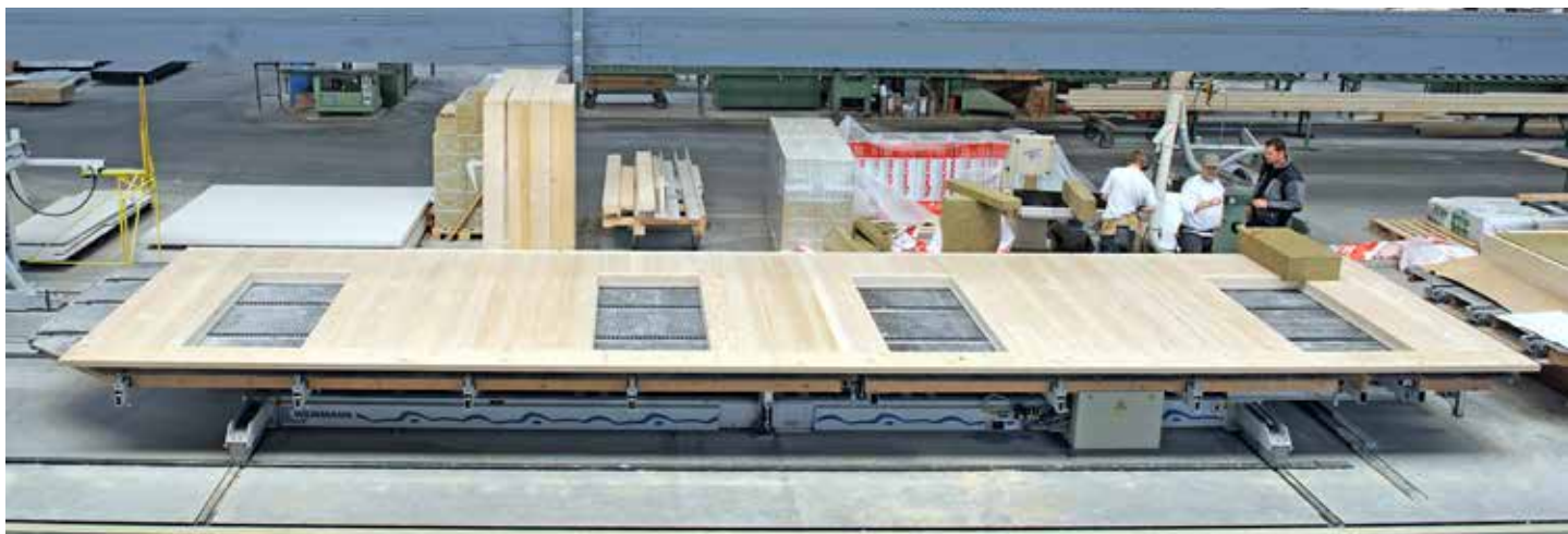
Wall panel fabrication for Holz8 Photo credit: Huber&Sohn
